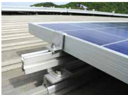
Figure 3: PV panel mounting structures
