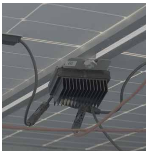
Figure 35: DC Optimiser installed under a PV panel
