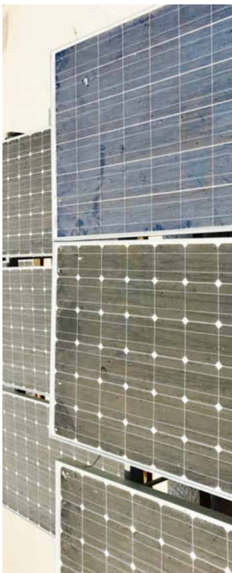
Figure 36: System with both mono and polycrystalline PV panels
