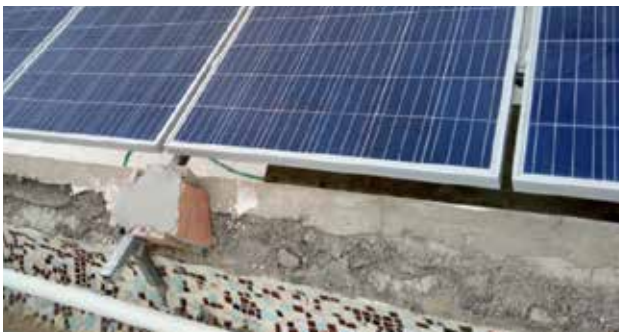
Figure 38: Mounting structures installed inadequately
