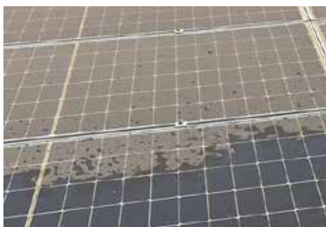
Figure 26: PV panel with dust accumulation
