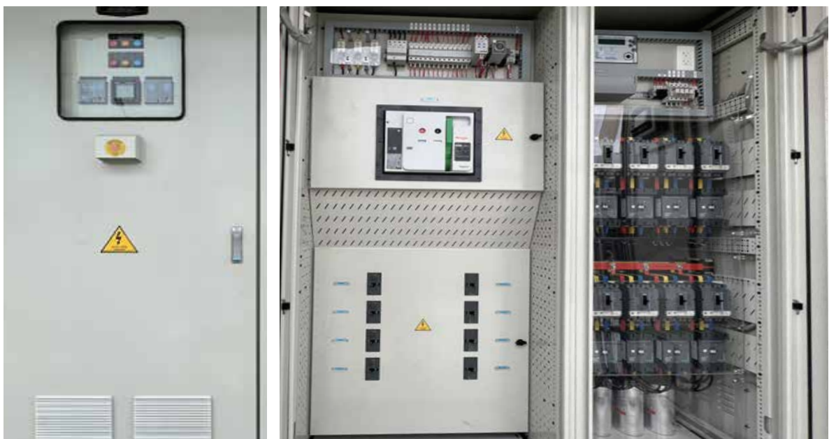
Figure 6: Outside and inside the AC distribution board
