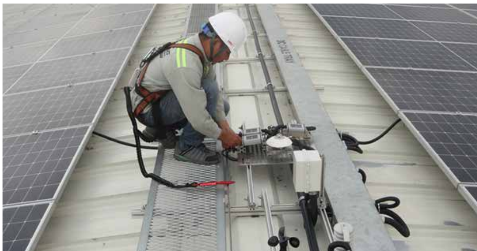
Figure 53: Workers are fully equipped with safety belts when working on a roof
