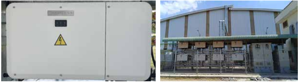
Figure 5: Inverter and inverter placement
