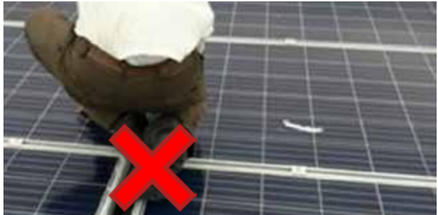
Figure 31: Do not climb, sit, or stand on PV panels
