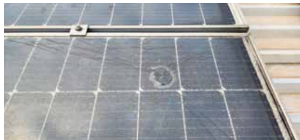
Figure 37: Examples of physical damage on PV panels
