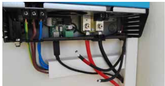
Figure 42: Cable detached from inverter
