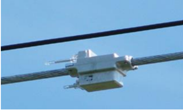
Figure 7: Line sag measurement modules from Belgian based company Ampacimon, installed at transmission lines of the Belgian TSO elia. The modules allow a continuous calculation of the maximum permanent flow that the line is supporting. [14]
