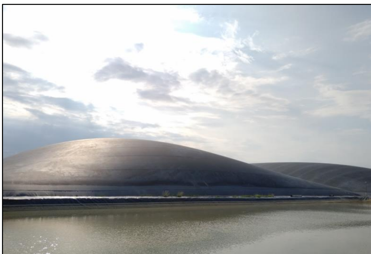
Figure 31: Biogas plant of Hung Duy Tapioca Starch factory
