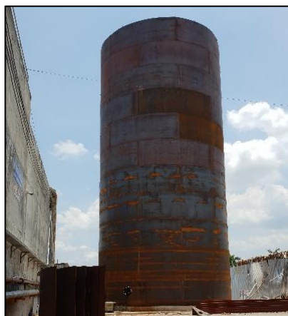
Figure 14: Anaerobic digester at Dong Tien paper factory
