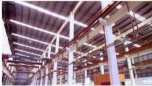
Figure 17. Day lighting with poly carbonated sheets
